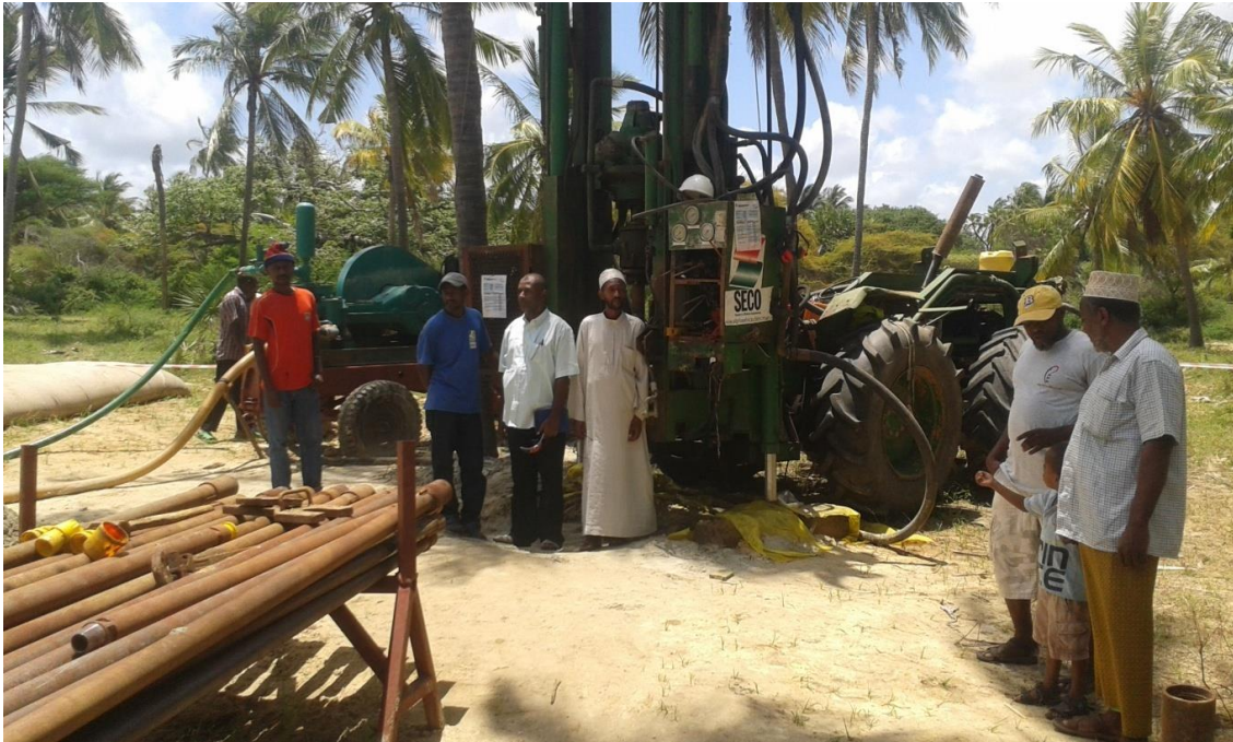
Figure 5.57. Water well drilling at Siyu
