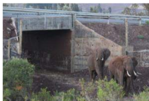
A typical underpass that allows animals to pass through under the road
