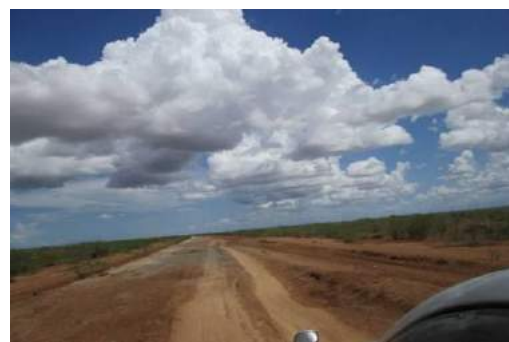
Portion of B8 - Hola to Bura West with Poor Condition of Road Due to Inadequate Drainage
