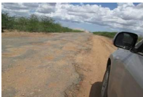
Portion of B8 - Hola to Bura West with Poor Condition of Road Due to Inadequate Drainage
