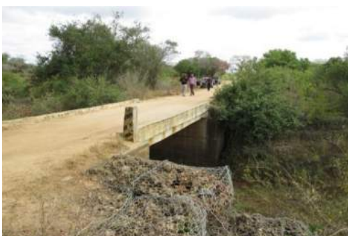
Minor Bridge parallel to Km 20/000 1 Span of 8.0 m
