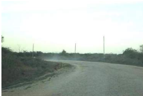
Poor Geometry on B8 Road
