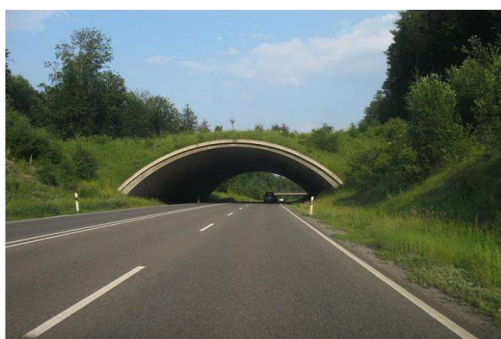
A typical overland crossing bridge (should have fencing that serves to funnel wildlife toward passage structures)
