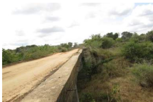
Minor Bridge parallel to Km 35/000 2 Spans of 10.50 m
