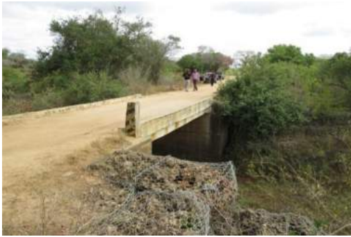
Minor Bridge Parallel to Km 21/000 1 Span of 8.0 m
