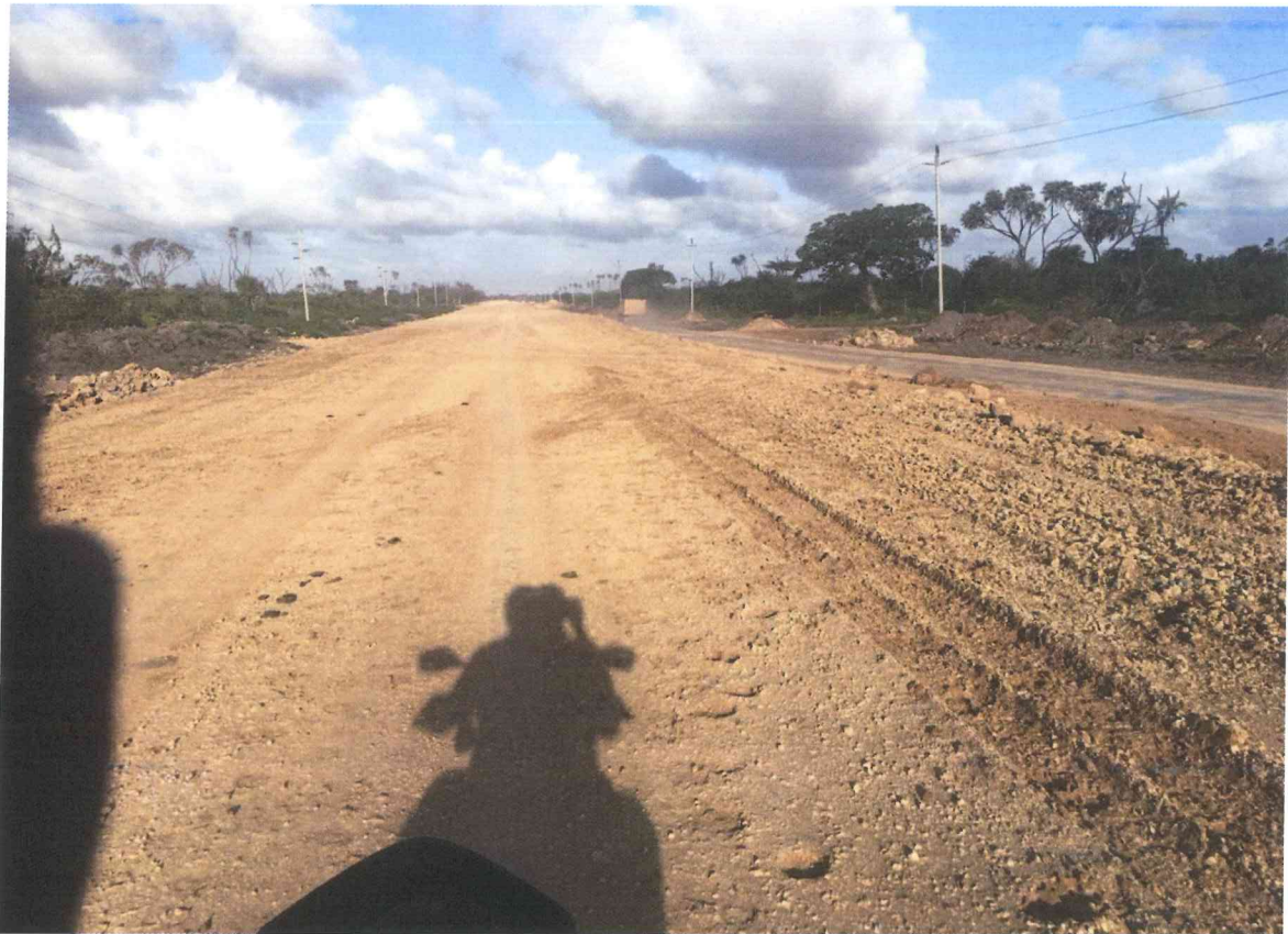
Figure 4: Photo showing the on-going road construction at the project site
