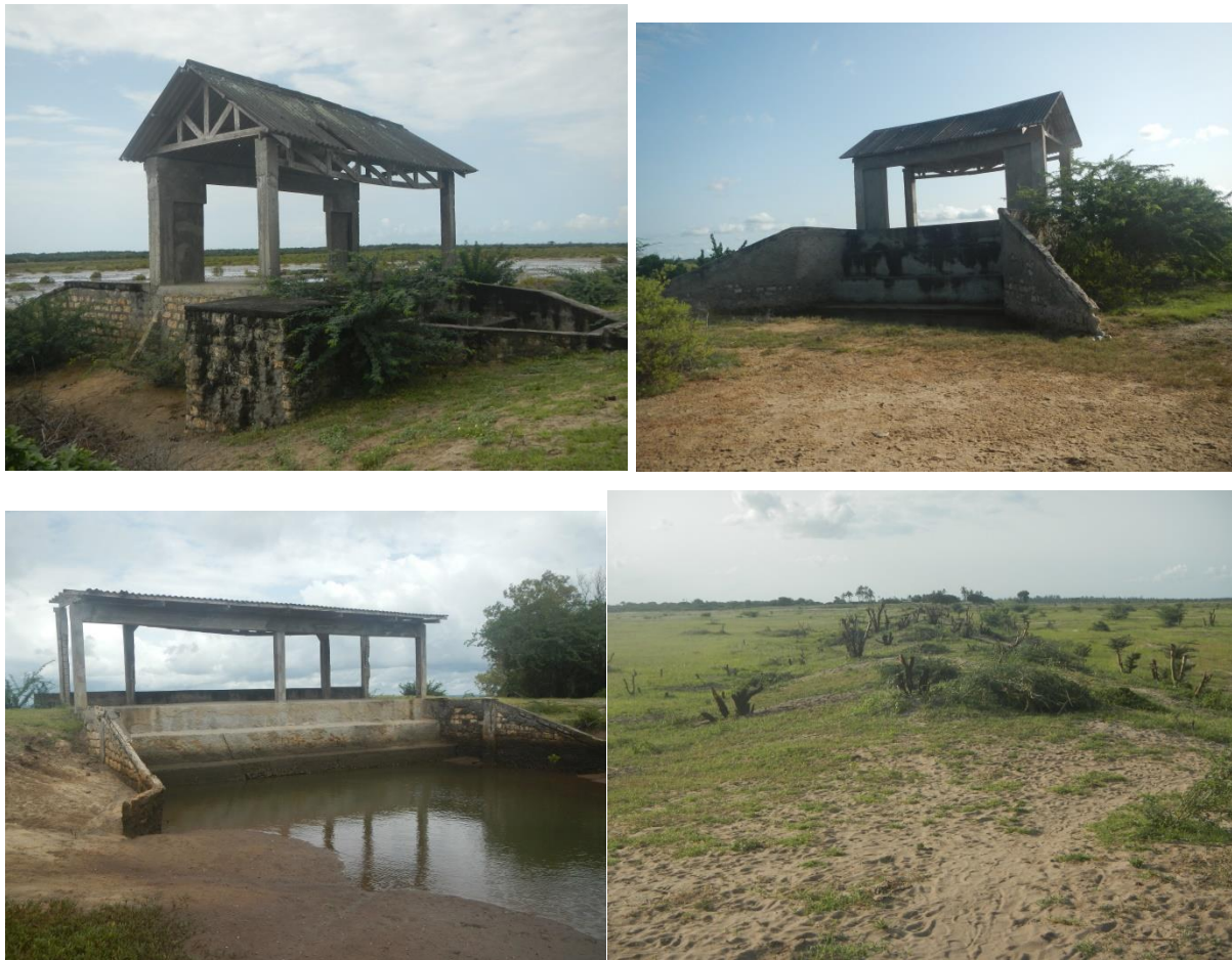
Plate 1: Remnants of pump station 3, 2 & 1 and one of the disintegrating dykes on site
