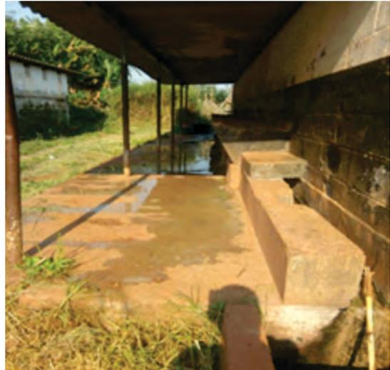
**Figure 7: Redwing mine toilets flowing raw sewage**
