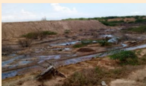
Illegal expansions and continued violations of law have seen important water sources for local community destroyed. Natural Justice is supporting community environmental legal officer teams who are undertaking environmental audits to ascertain project impacts and monitor legal compliance.
