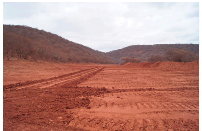
Marsabit County, Kenya - Highway being built.
